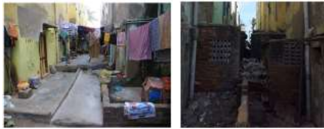
Fig. 12. Encroachment on the front yard of the blocks b. Encroachment behind the housing blocks
