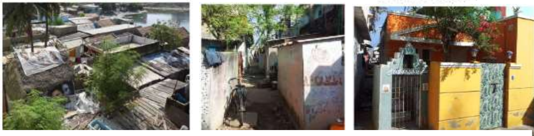
Fig. 11 Encroachment on back waters b. Encroachment along G+1 blocks c. Pucca structure built on encroached land next to G+1 Block.
