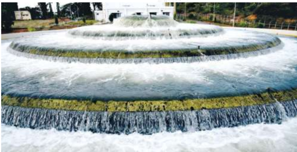
Figure 1 : CASCADE AERATOR
