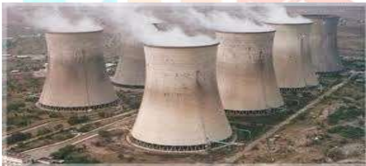
COOLING TOWERS, RTPS PHOTO—3.9
