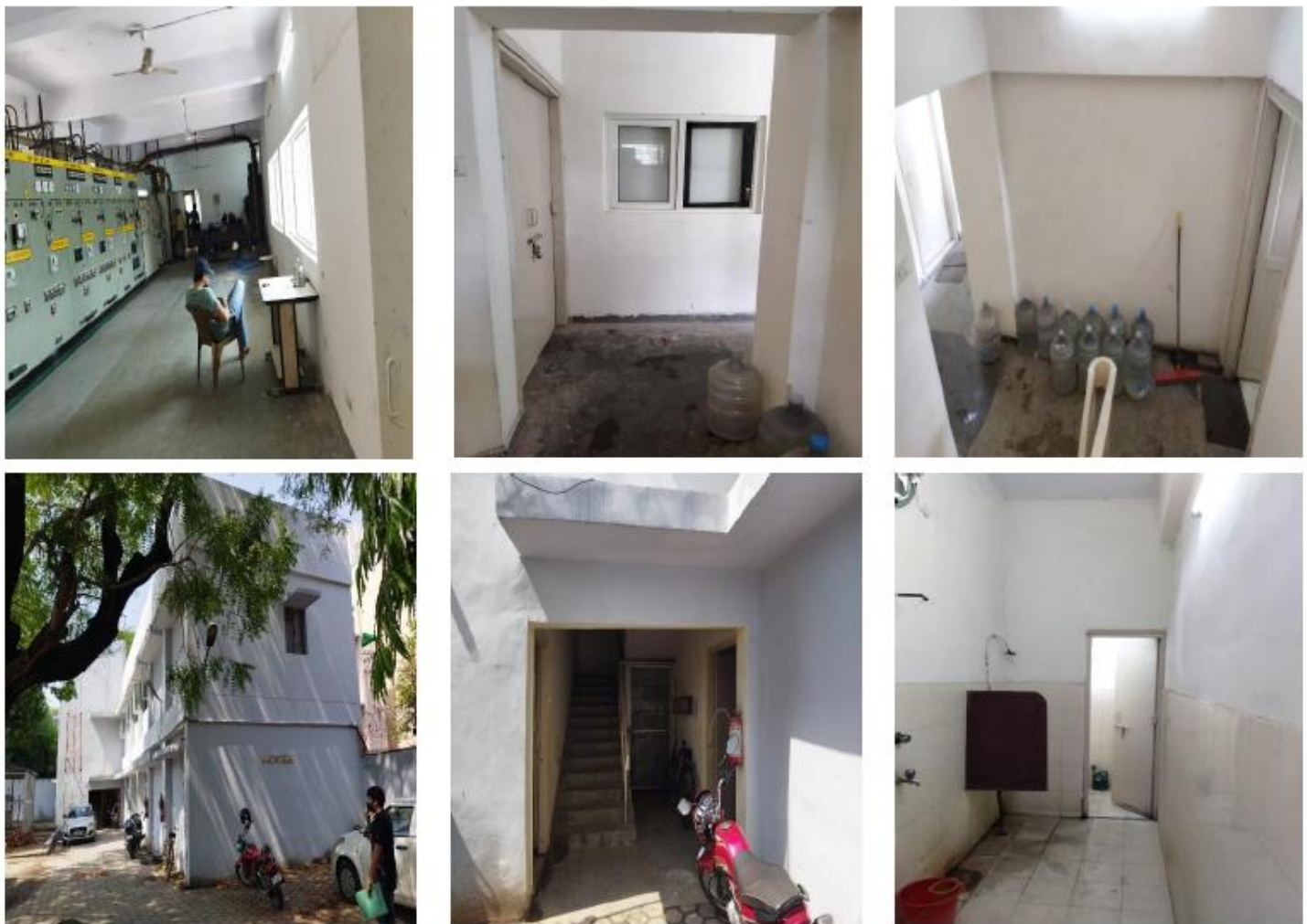
FIG: 9 SHOWING NO DISTRESS.
