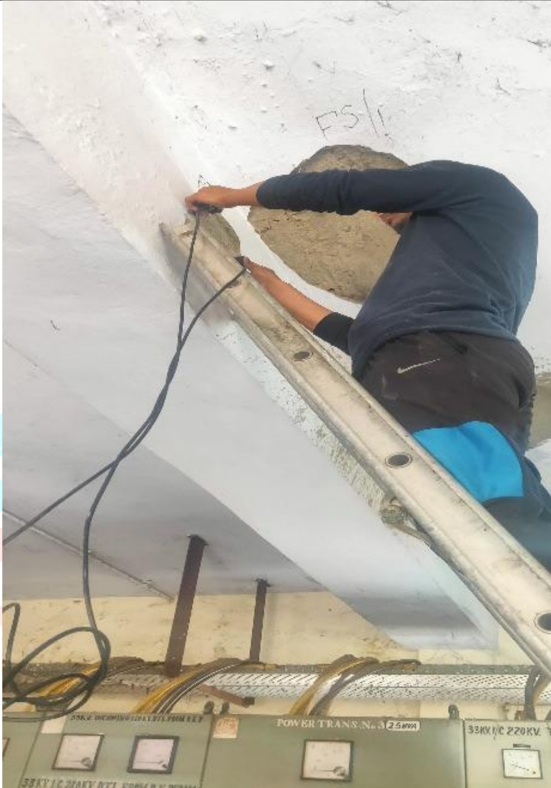
FIG:4 UPV TEST IN PROGRESS BHIKAJI KAMA GRID
