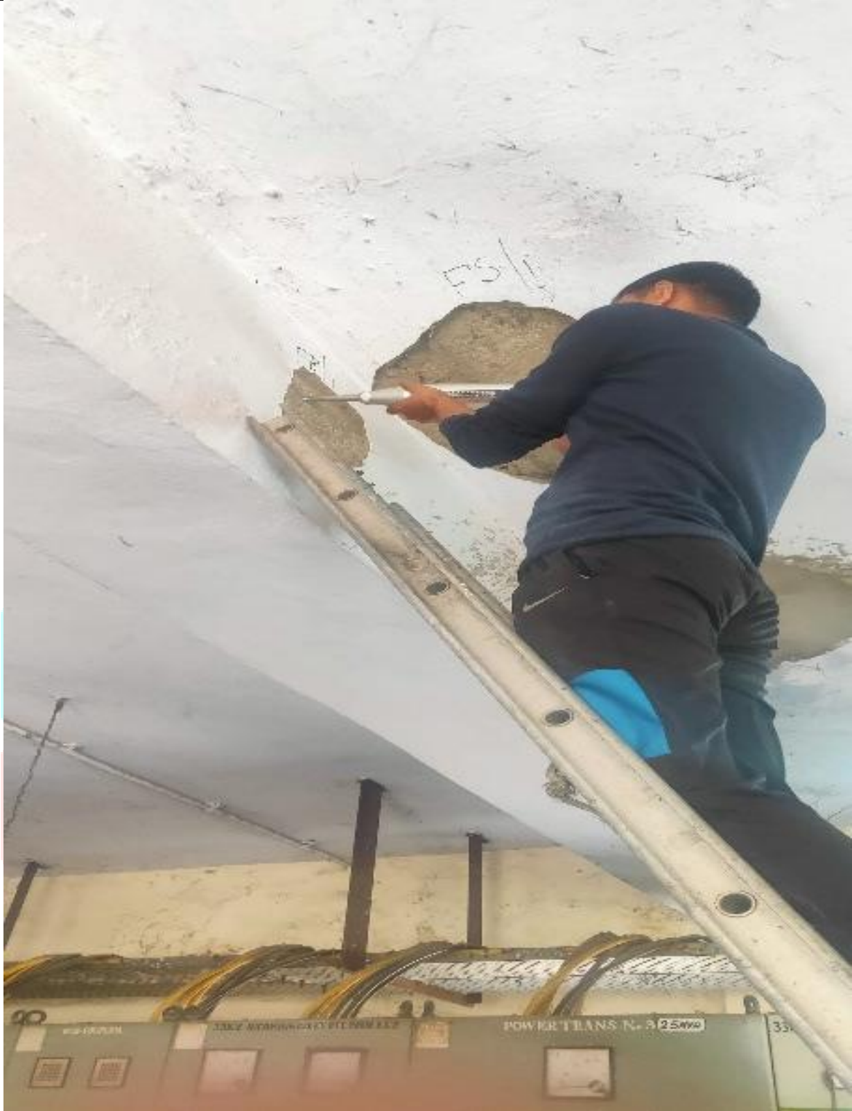
FIG: 7 RBH TEST IN PROGRESS
