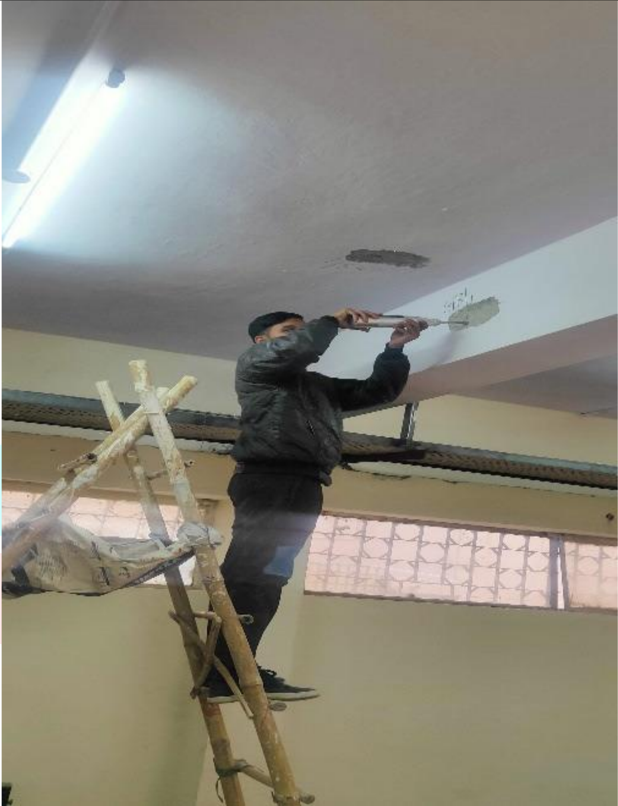
FIG: 6 RBH TEST IN PROGRESS
