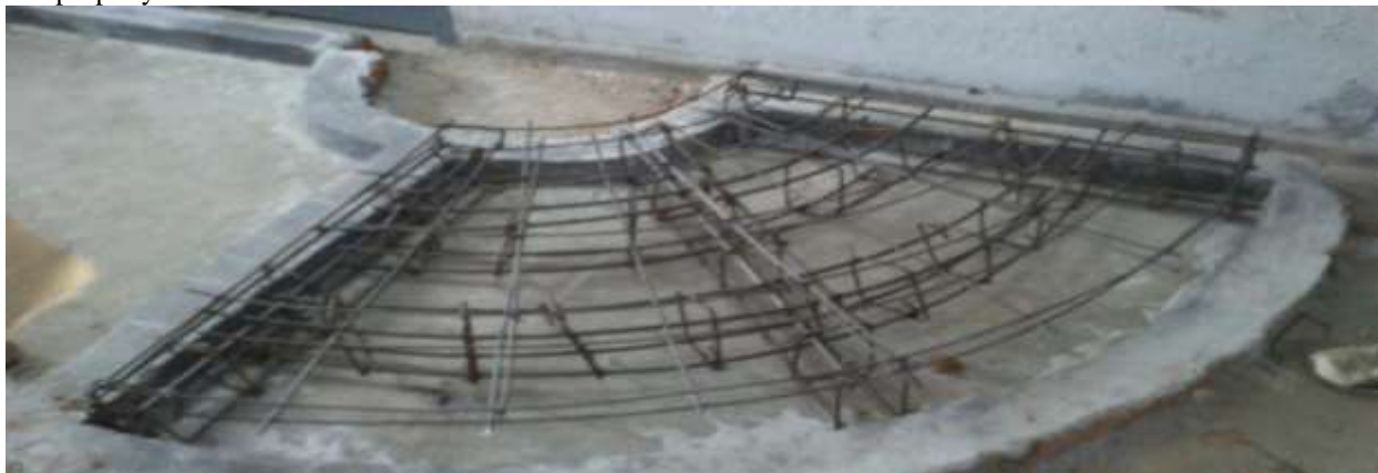
Fig 3.2.2: Reinforcement mesh
