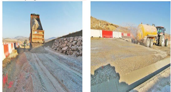
Figure 7 Delivery and Watering of CDW aggregate to the jobsite
