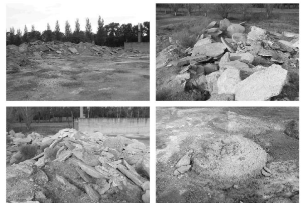
Figure 3 Deposit of remains of ready-mix concrete in a concrete-manufacturing company
