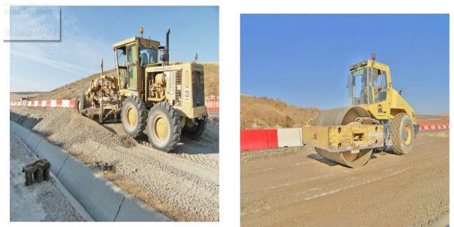
Figure 8 Spreading and layer CDW aggregate to the jobsite
